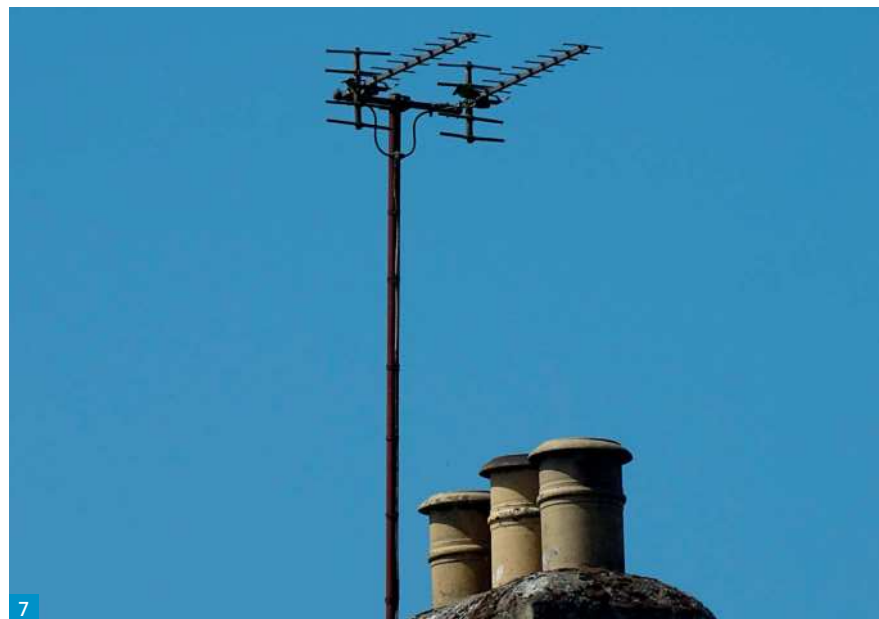
Fig. 1: A 3-element Yagi beam for FM radio, atop a small Yagi for TV. Fig. 2: Basic arrangement of a 4-element Yagi antenna. Fig. 3: Signal spread from a small Yagi antenna. Fig. 4: Signal spread from a long Yagi antenna. Fig. 5: Signal spread from two stacked Yagi antennas. Fig. 6: Signal spread from two bayed Yagi antennas. Fig. 7: Bayed TV antennas, to give a narrow beam.
